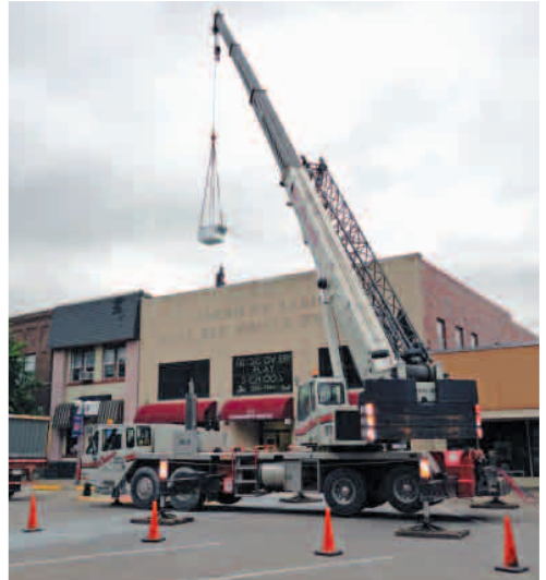
Setting mechanical equipment
