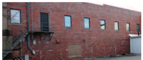
New storm windows
