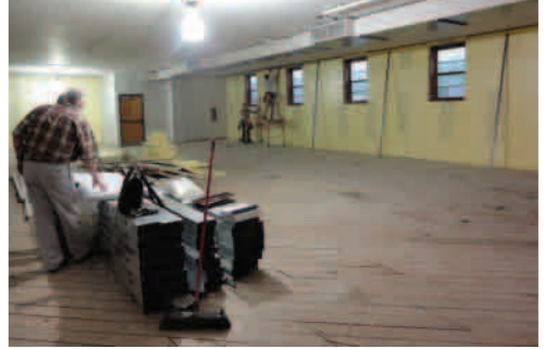
Adding wall insulation
