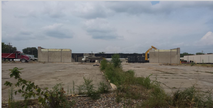
Construction site of Fareway
