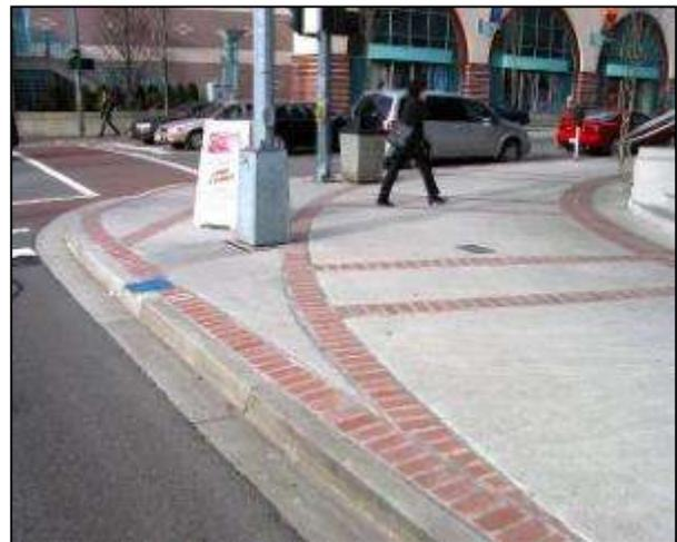
*Figure 8. Reducing the radius of a turn reduces traffic speed and greatly improves safety for bicyclists and pedestrians.*
