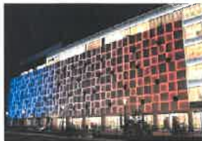
ARCHITECTURAL FACADE LIGHTING
