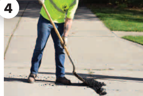
SHOVEL IN HOT MIX ASPHALT
