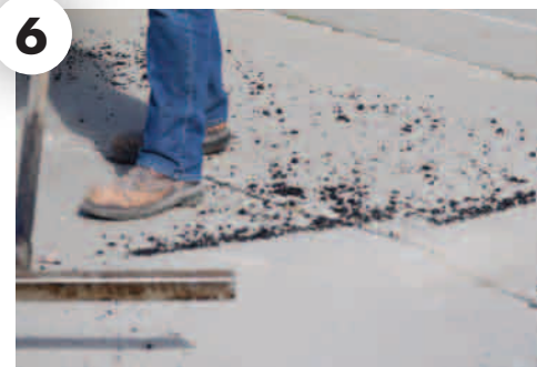
CLEAN THE AREA
