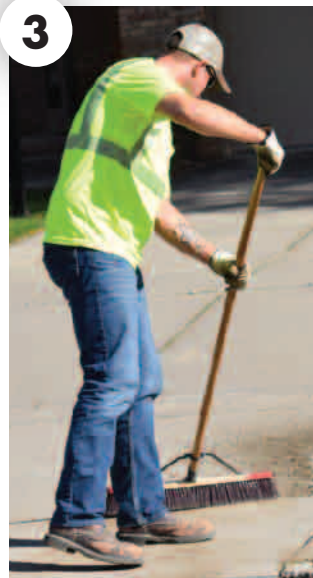
CLEAN THE AREA
