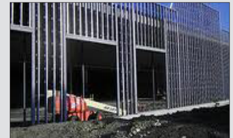
Construction site of Whole Foods
