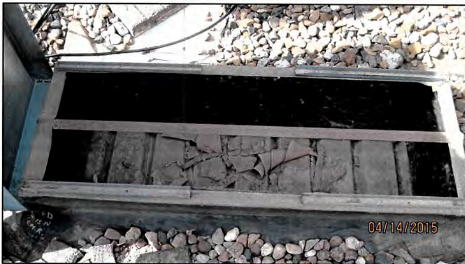
Figure 15: East Elevation, vacant mechanical curb. Roof curbs and penetrations should be capped below the new system to reduce roof penetrations.
