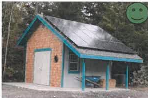
Correct: Panels are within 1 foot of roof surface
