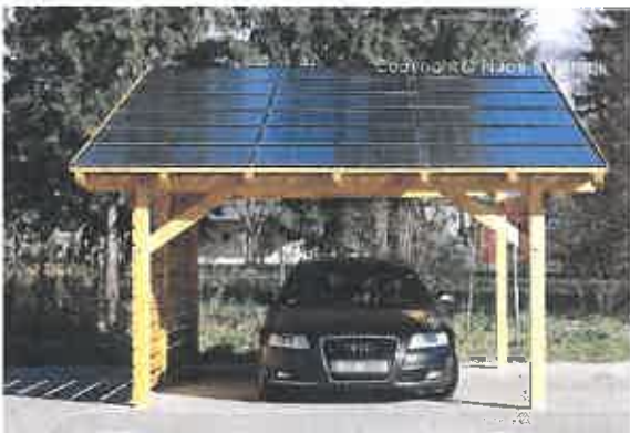
Detached structure – Residential carport
