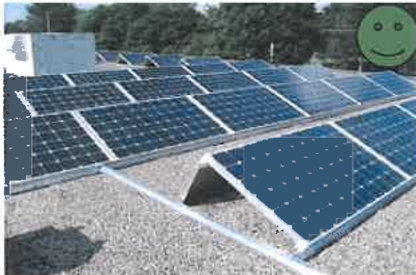
Correct: System height less than 7' above roof
