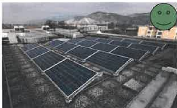
Correct: Panels are installed far from roof edge no fall protection rail required
