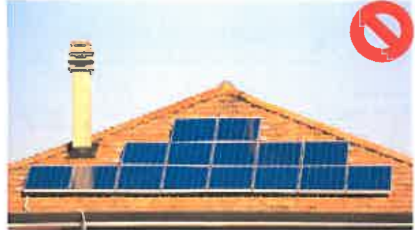
Incorrect: Inconsistent arrangement, does not follow the shape of roof
