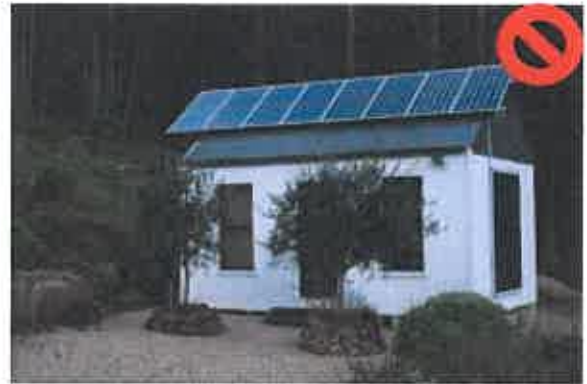
Incorrect: Panels extend past the roof edge
