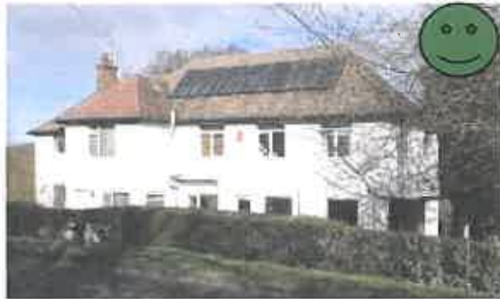
Correct: Consistent arrangement and centered in the available roof area (does not need to match shape of roof)
