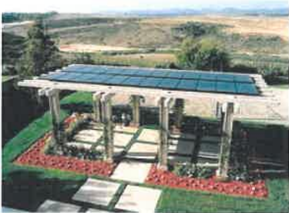
Detached structure -Trellis or pergola
