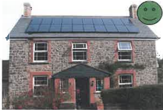
Correct: Panels are setback from roof edge and have access aisles
