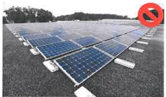
Incorrect: Frame and equipment do not match roof color
