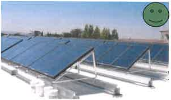
Correct: Frame and equipment match roof color
