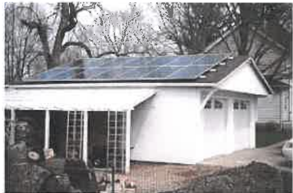
Detached structure – Garage
