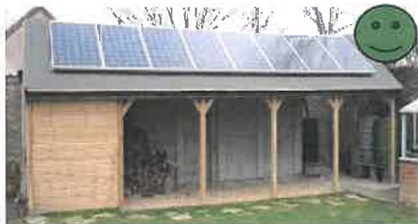
Correct: Consistent arrangement, no gaps
