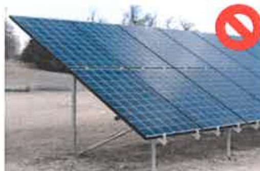
Incorrect: No screening of framework
