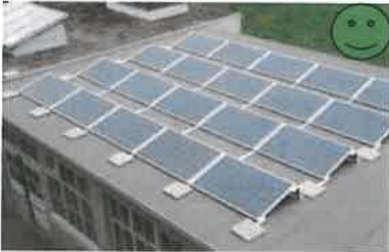
**Correct: Consistent arrangement, no gaps matches roof proportions**
