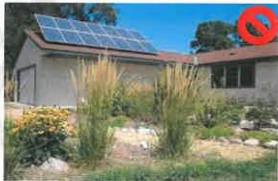
**Incorrect:** Panels are mounted higher than 1 foot from roof surface
