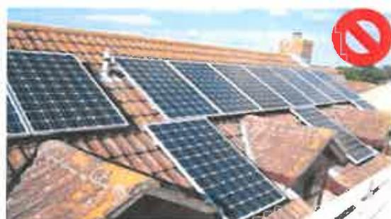
Incorrect: Not consistent, gaps in arrangement
