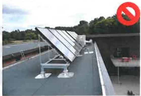
Incorrect: System height greater than 7' above roof
