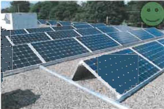
Correct: System height less than 7' above roof
