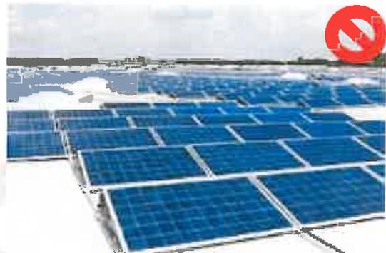
**Incorrect: Not consistent, gaps in arrangement**
