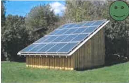
Correct: Framework enclosed in materials compatible with primary structure
