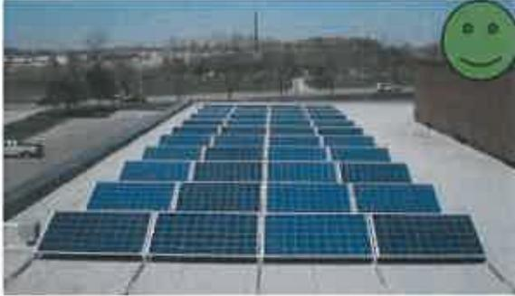
Correct: Panels are set back from roof edge
