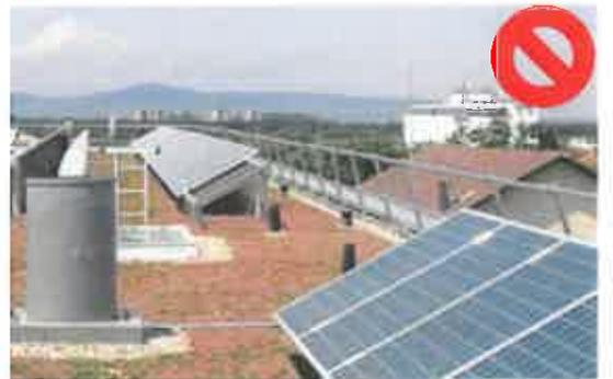
Incorrect: Panels are installed close to roof edge requiring a fall protection railing
