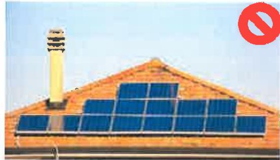
Incorrect: Inconsistent arrangement, does not follow the shape of roof
