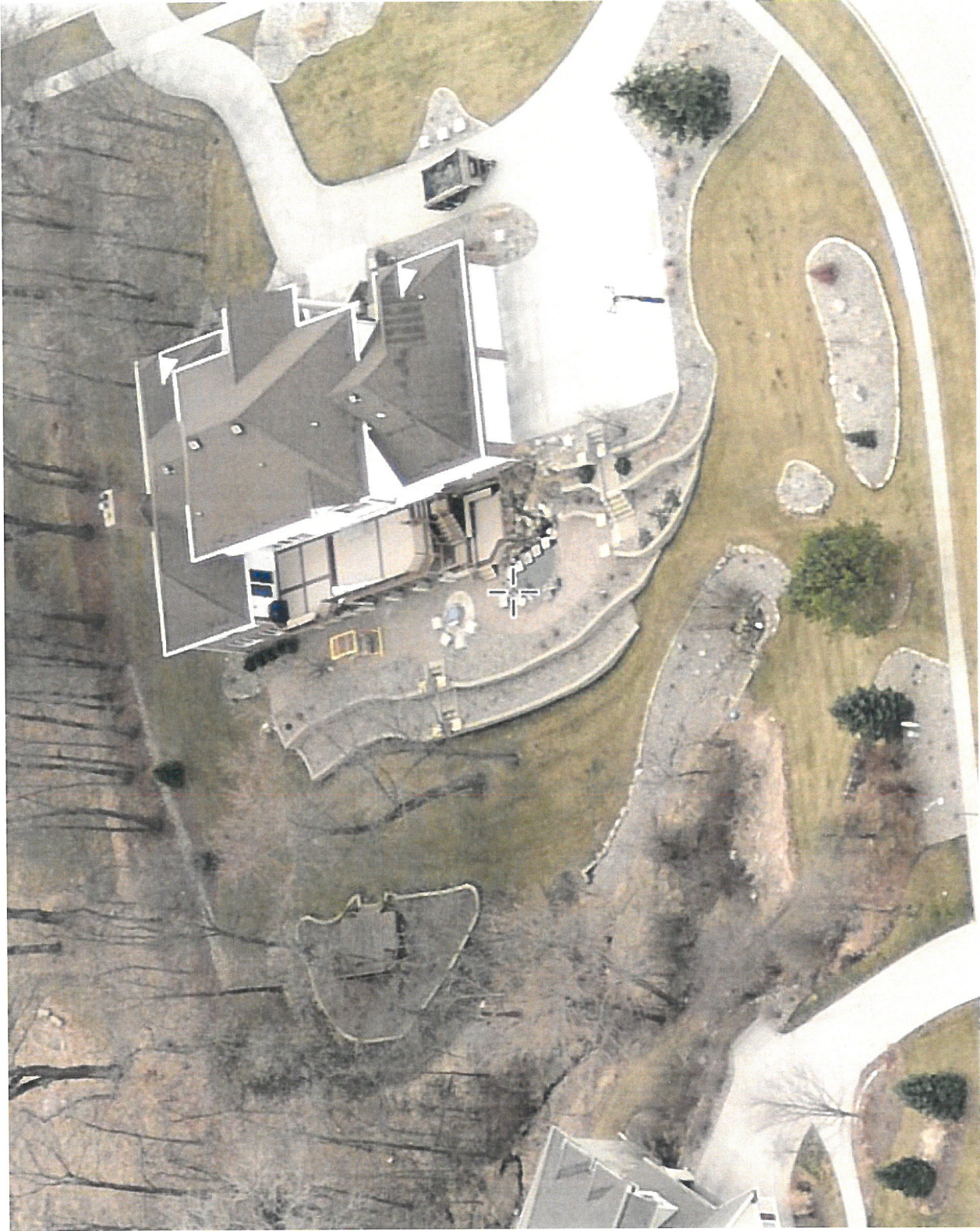
North Looking South
