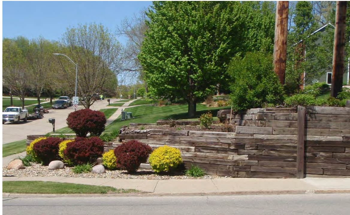
EAST OF 33rd ST. - LOOKING NORTH WEST RETURN
