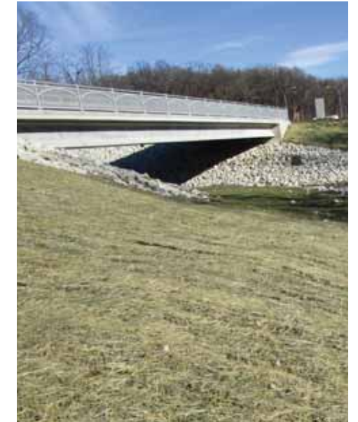
Stagecoach Drive Bridge
