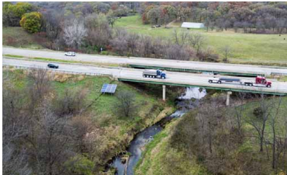
TOP: North half of project area from Woodland Hills facing north toward Interstate 80 (not visible). BOTTOM: The trail will pass under I-35 into the City of Waukee at the north end of the project.
