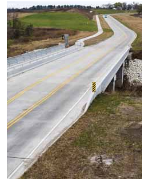
Grand Prairie Parkway Bridge
