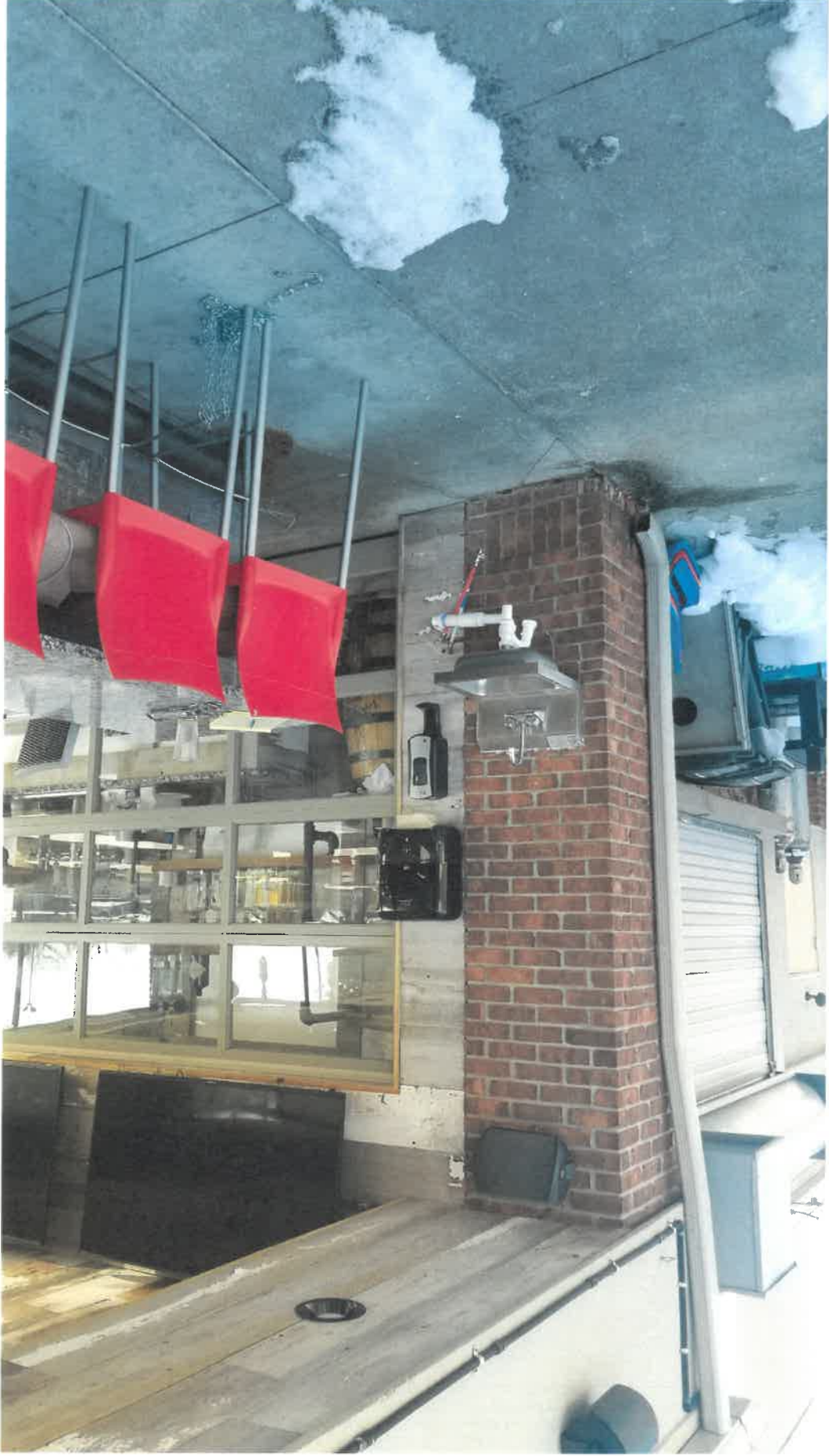
CLOSE UP VIEW OF NORTH SIDE OF EXISTING STRUCTRE
