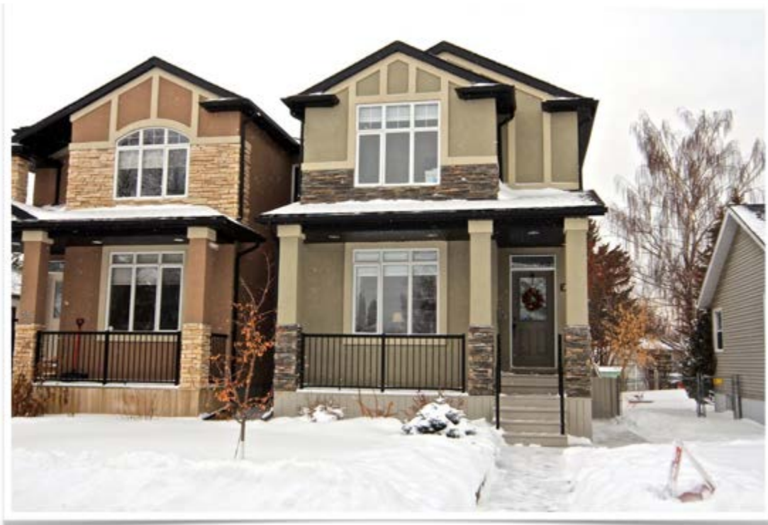
17 feet wide single family homes on 25-foot-wide lots are a common Inner City building form in Calgary, Alberta. These two houses have replaced a one story single family home on the original 50-foot lot.
