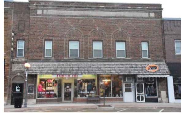
EXISTING BUILDING FACADE
