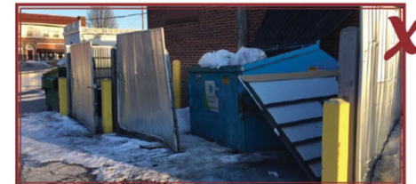
A trash enclosure not constructed of durable, cohesive materials. Credit: City of West Des Moines
