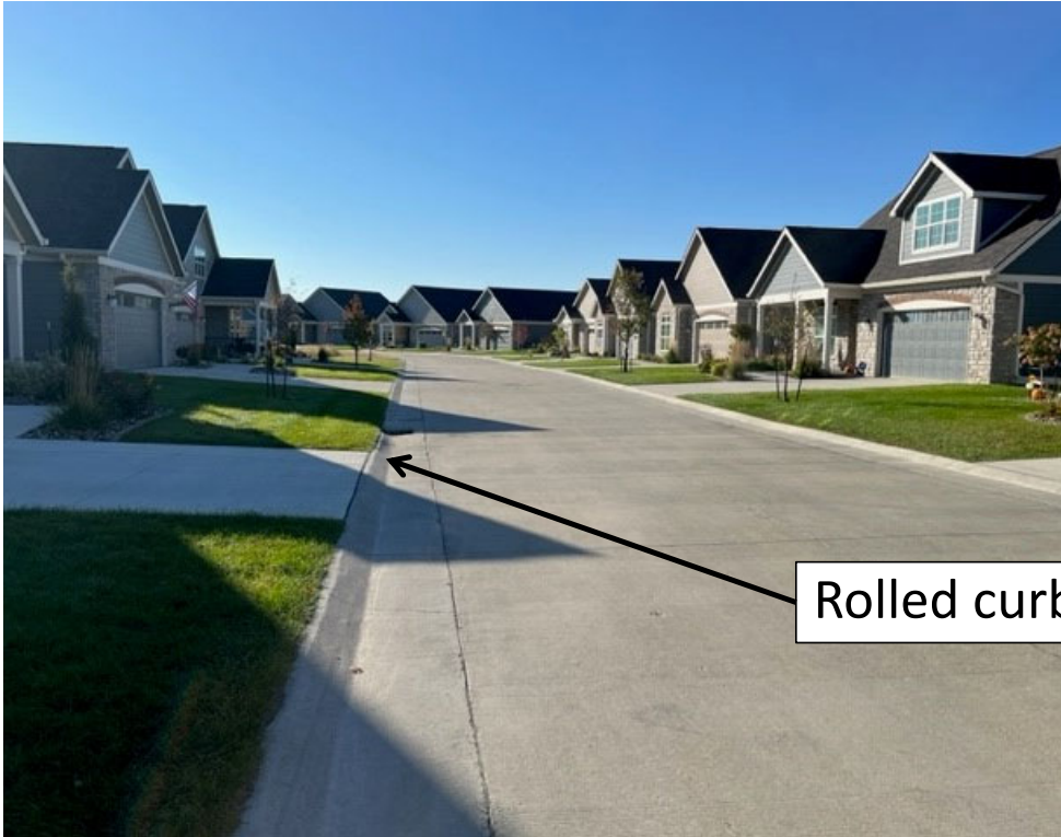
Rolled curb, no sidewalks
