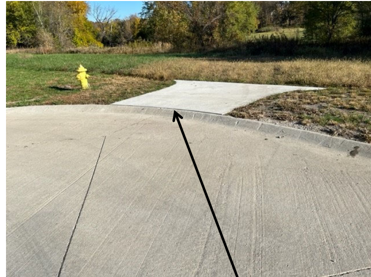
Rolled curbs are not accessible
