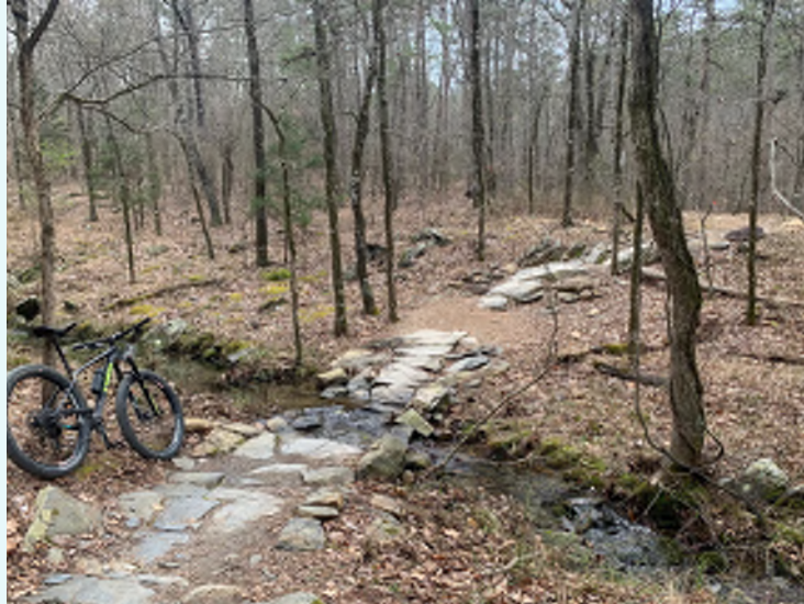
TECHNICAL FEATURE: ROCK ARMORING
