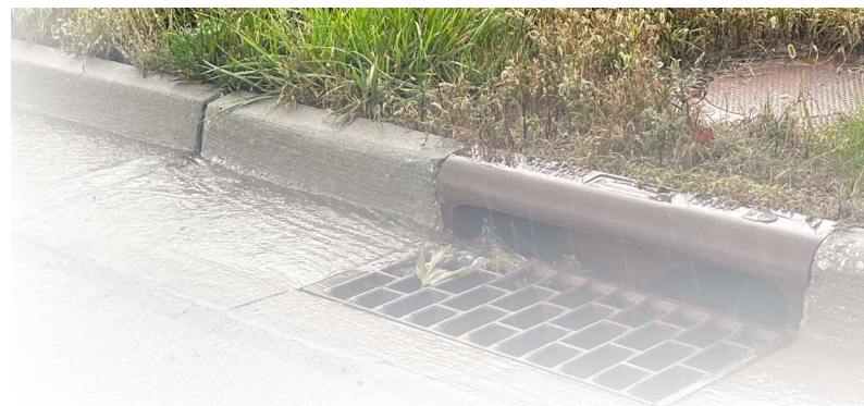
Stormwater drains off landscapes into street inlets connected to an underground stormwater sewer pipe system.
